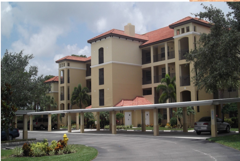
Island Sound II Bldg
